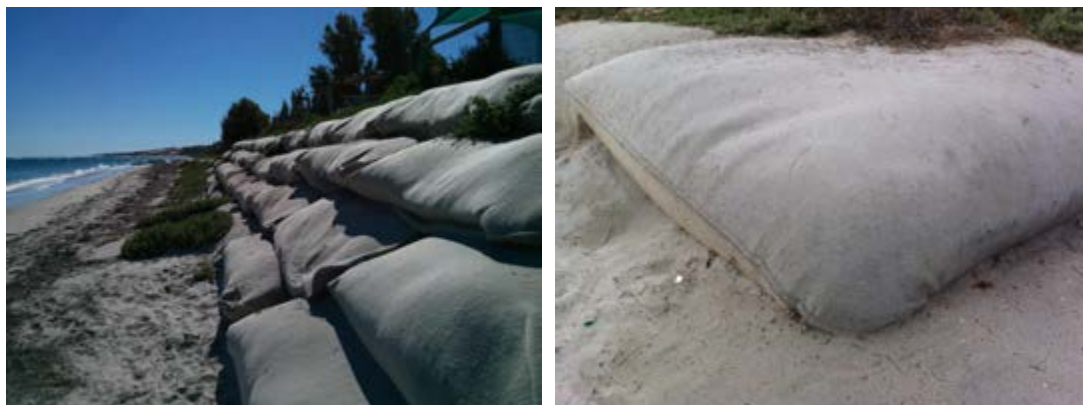
Plate 25: Geotextile shoreline protection at Horrocks Beach
