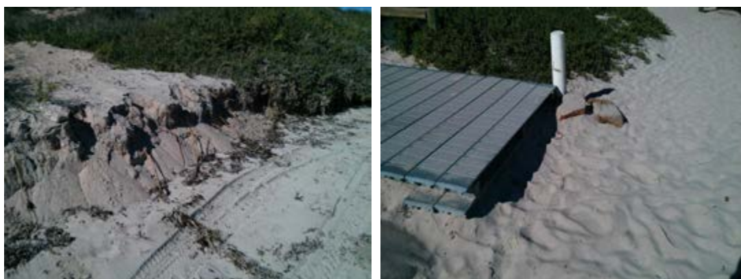
Plate 18: Erosion from coastal processes at Horrocks Beach
