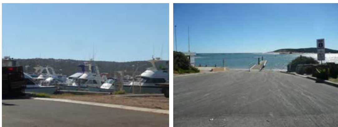
Plate13: Kalbarri Marina and Jetty Facilities
