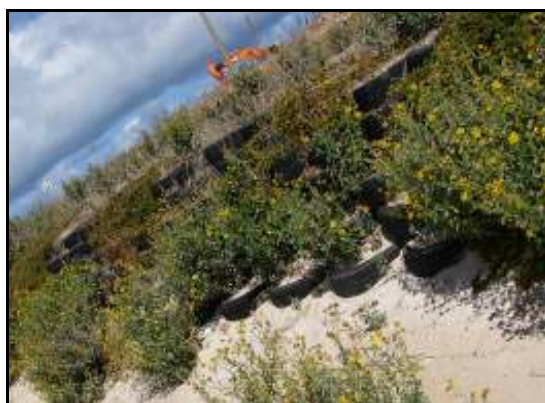
Photo 4.4: Tyre bunding wall at the Dongara Transfer Station (Shire of Irwin)
