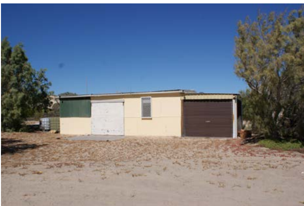
Photo 4: Cottage, Halfway Bay (Land Insights 2016)
