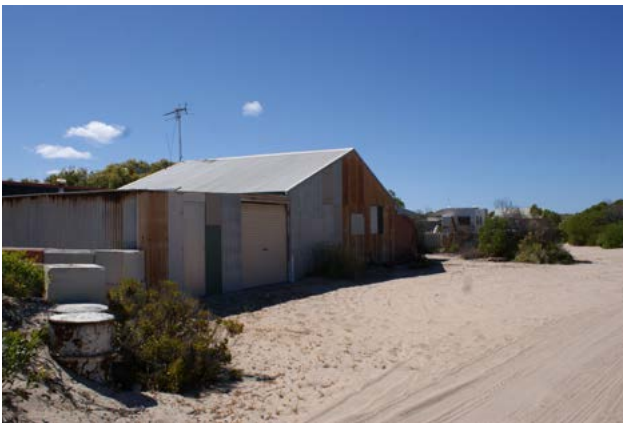
Photo 3: Cottage, Halfway Bay (Land Insights 2016)
