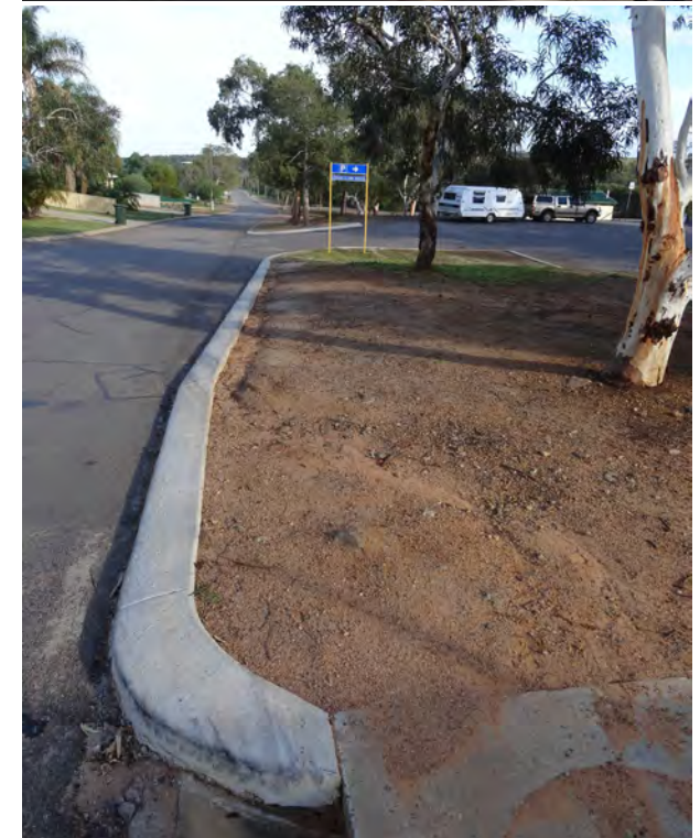
Above: Sections of the Main Street and roads leading out of the main street do not have continuous footpath treatments
