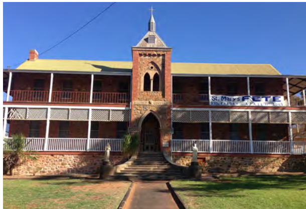
Above: The Old Road Boards Office and Old Convent, two of the historical buildings located on Northampton's Main Street
