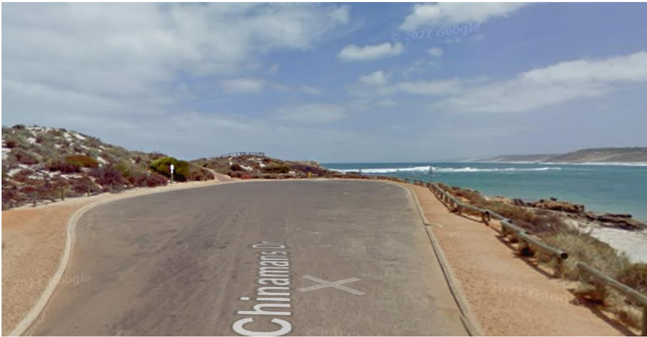
Photo 3 Sealed car park before the impact of STC Seroja
