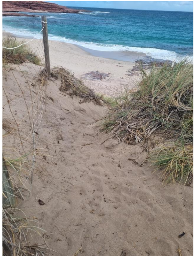
Photo 6 Damaged fence and posts to be reinstated
