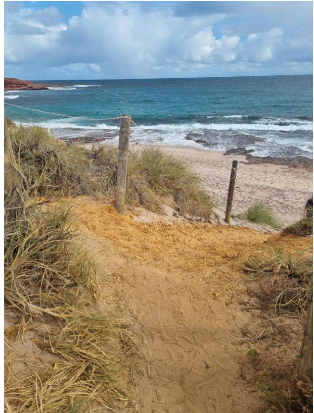
Photo 4 Beach access – temporary works undertaken. Damaged fence and posts to be reinstated
