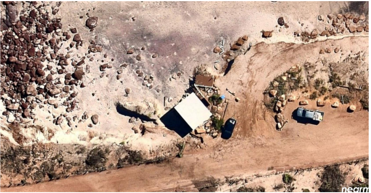
Photo 3 Damaged structure, emergency vehicle beach access and pedestrian beach access
