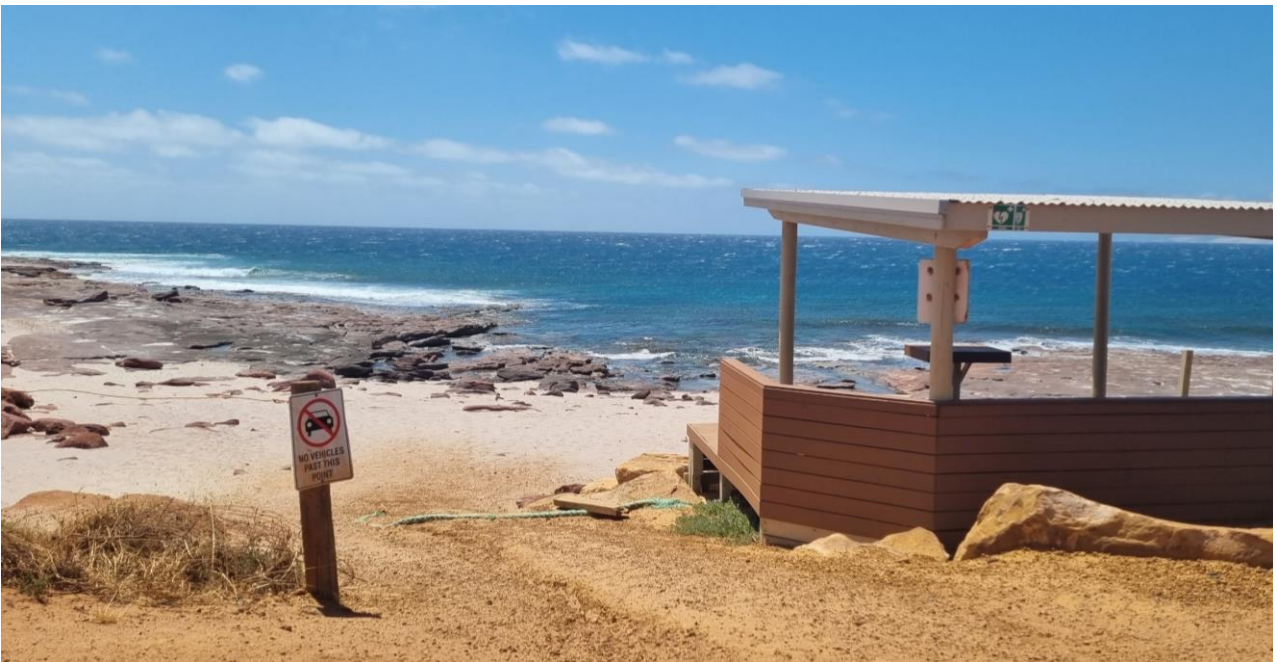
Photo 6 Emergency beach access and shelter damaged
