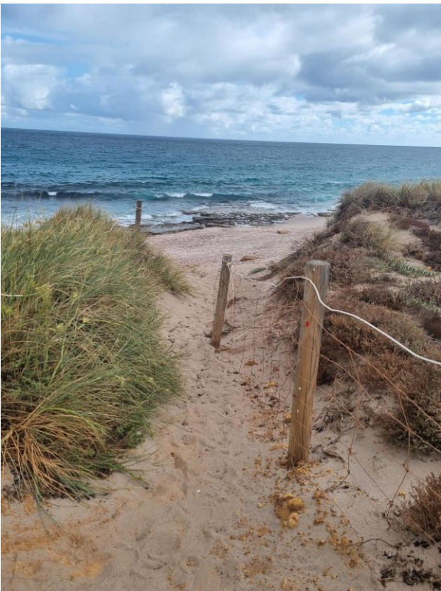
Photo 9 Damaged steel wire mesh fencing and path
