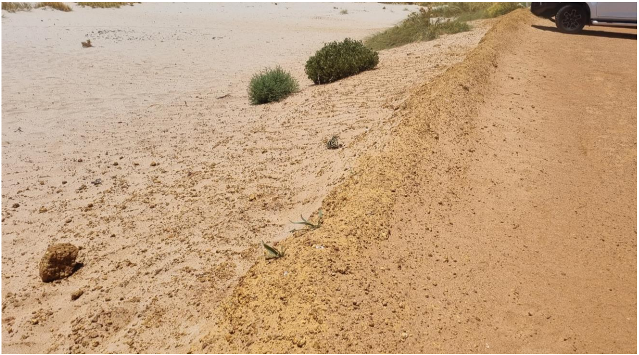
Photo 9 Damaged gravel car park
