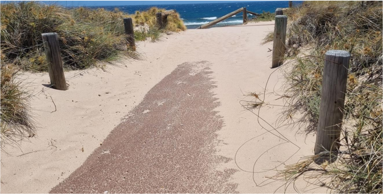
Photo 7 Sand to be cleared off the footpath and fencing to be reinstated
