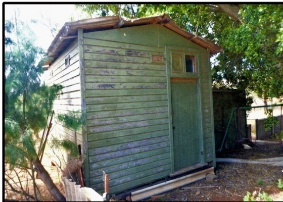
Photographs of Fettler's Hut and current condition
