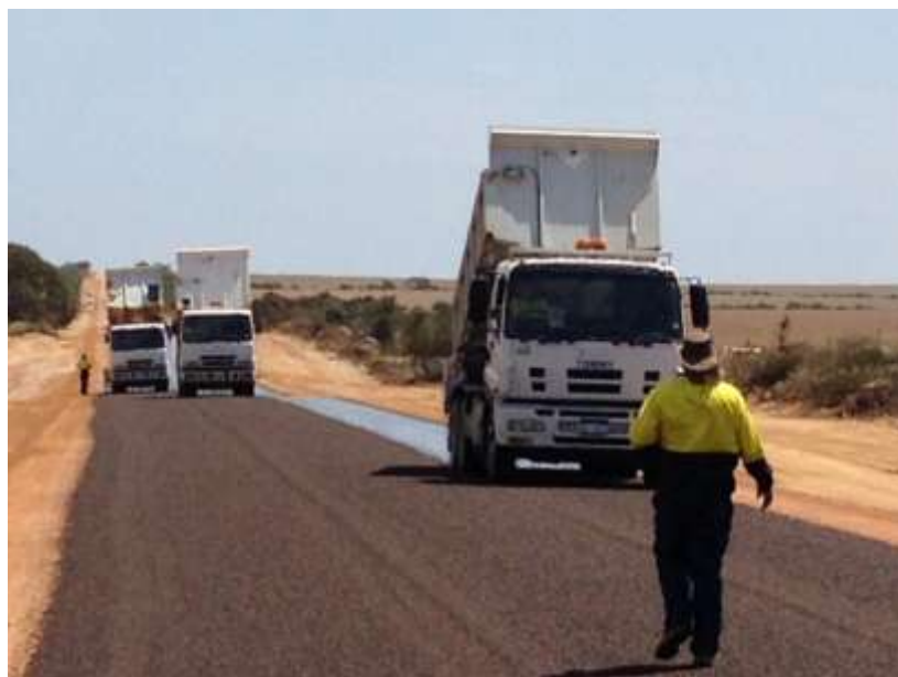
Sealing a section of Binu West Road
