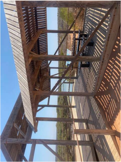
shark bay shade structures timber batten shade structures in shark bay protect from the sun whilst allowing air flow and rising hot air to escape
