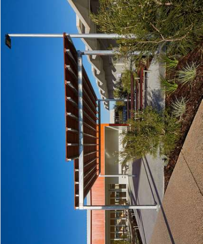
leighton beach facilities | bernard seeber architects timber battens on steel structure provides a robust materiality for coastal conditions
