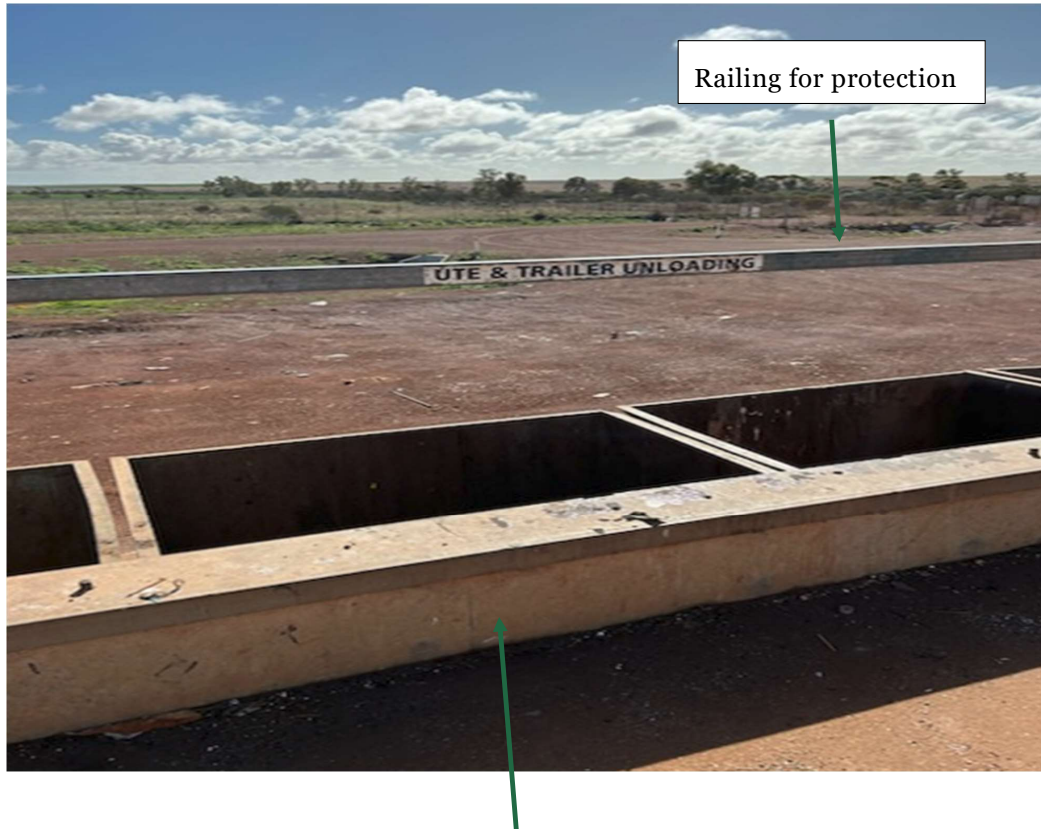
MULLEWA REFUSE SITE CONCRETE BARRIER FOR TRUCKS AND CARS TO REVERSE UP TO
