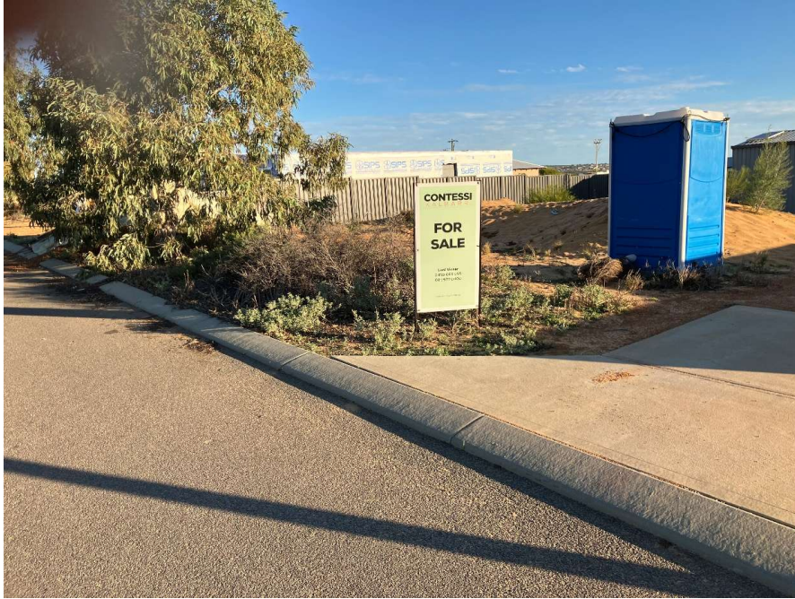
Builders Toilet abutting Front Boundary
