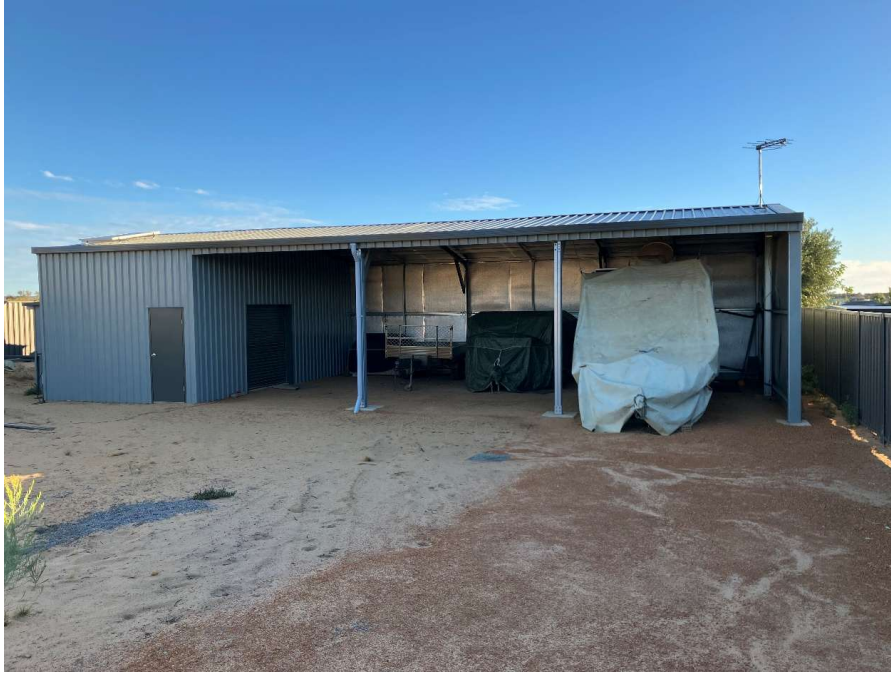
Approved Shed with Caravan, Camper and other trailer being stored. TV Antennae on right of roof, solar panels on left
