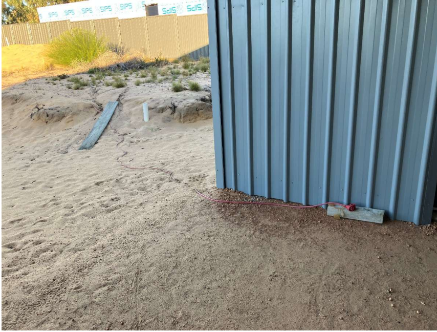
Power lead running from Builders Connection at front of the lot.
