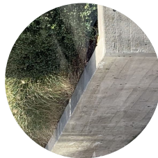
Retaining Walls (as required) Off-form reinforced concrete
