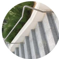
Stairs Concrete with SS handrails
