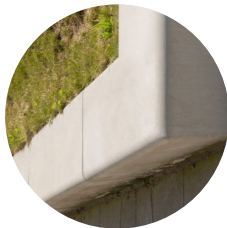
Seating Walls Off-form reinforced concrete
