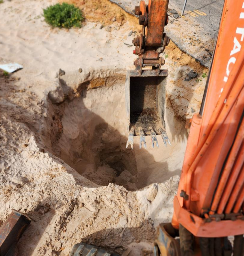
Figure 1 Chinaman's Beach - Test Pit – central location along work site
