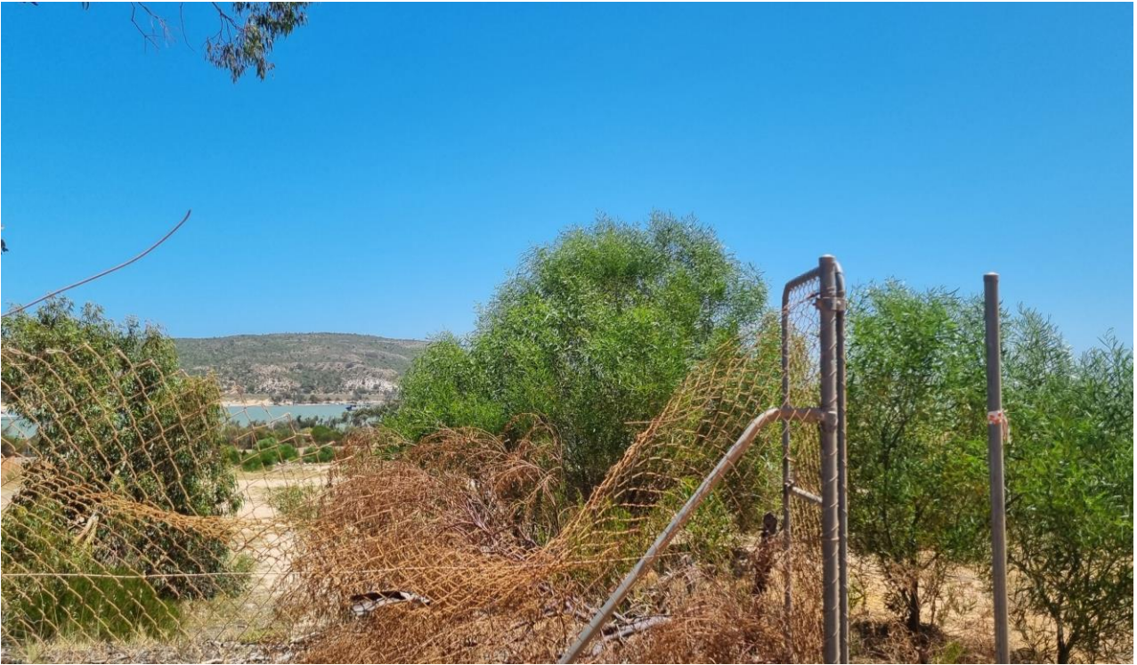
Photo 5 Existing fence to be repaired. New fence to tie in.
